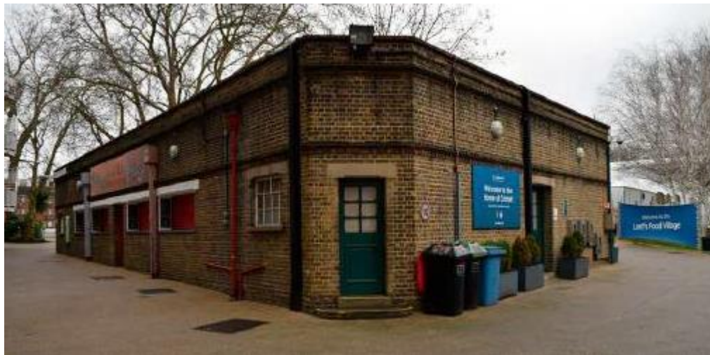
Full Toss Bar building from the South (to be demolished)
