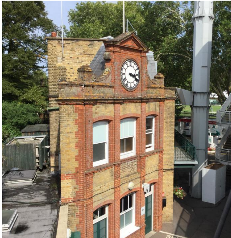
Clock Tower Building (to be demolished)
